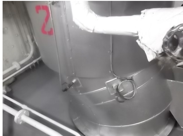
Figure 7 – Exhaust Stacks for DG1 (image at left) and DG2 (image at right)
