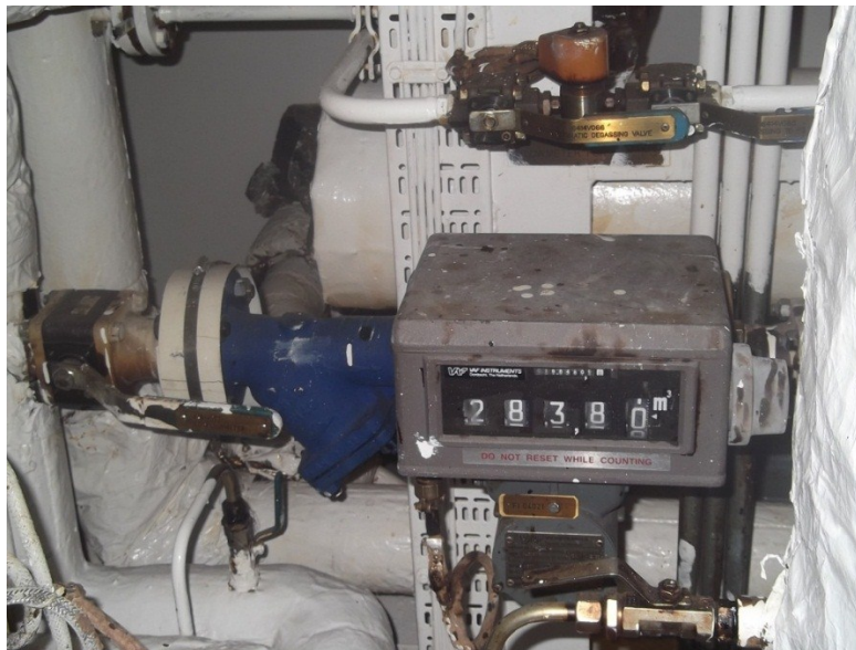
Figure 1 – VAF J5050 Flow Meter for Fuel Oil Consumption Measurements
