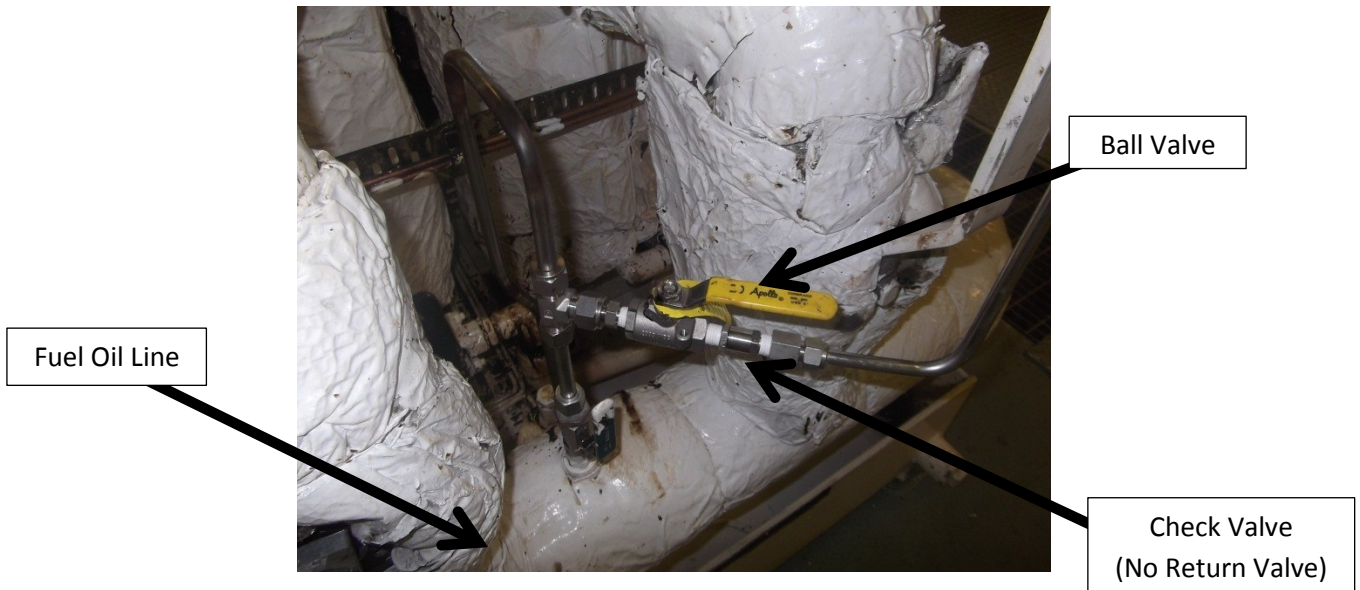
Figure 4 – FPC Injection Point
